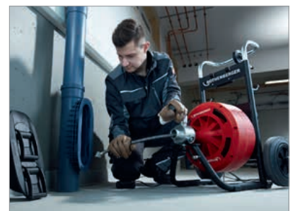
Cleaning of a down pipe with 16 mm spiral
