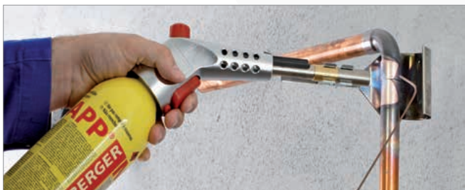
Brazing in gas installation
