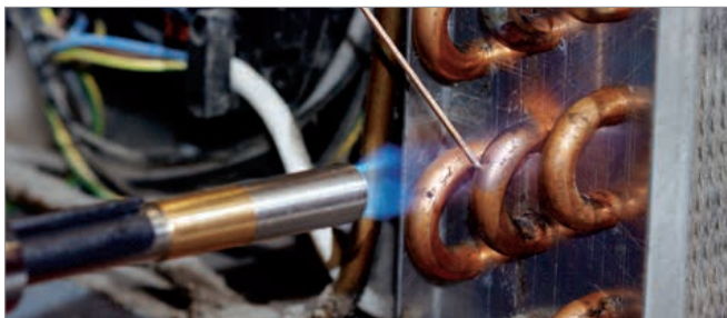
Brazing in aircon and refrigeration
